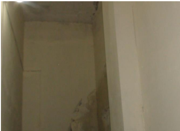
Dampness in Walls & Roof
