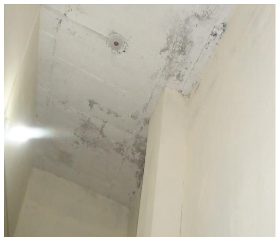
Dampness in Walls & Roof
