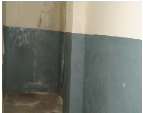
Dampness in Walls & Roof
